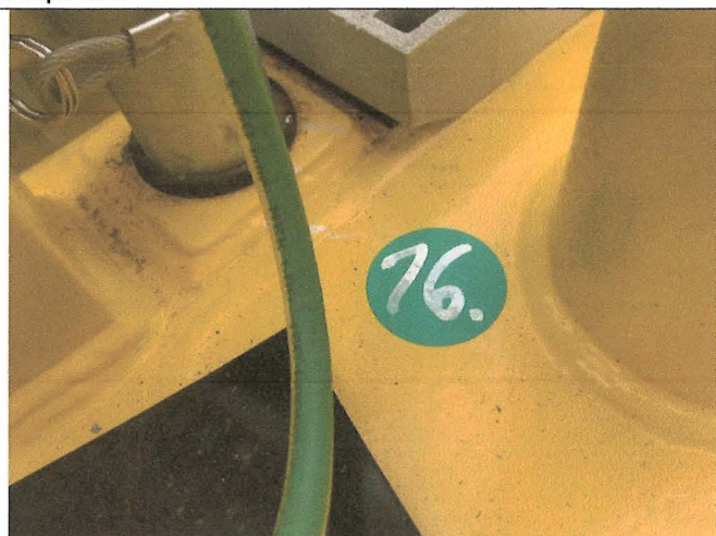
No. 16 - Dirt and fly rust. Cleaning required.
