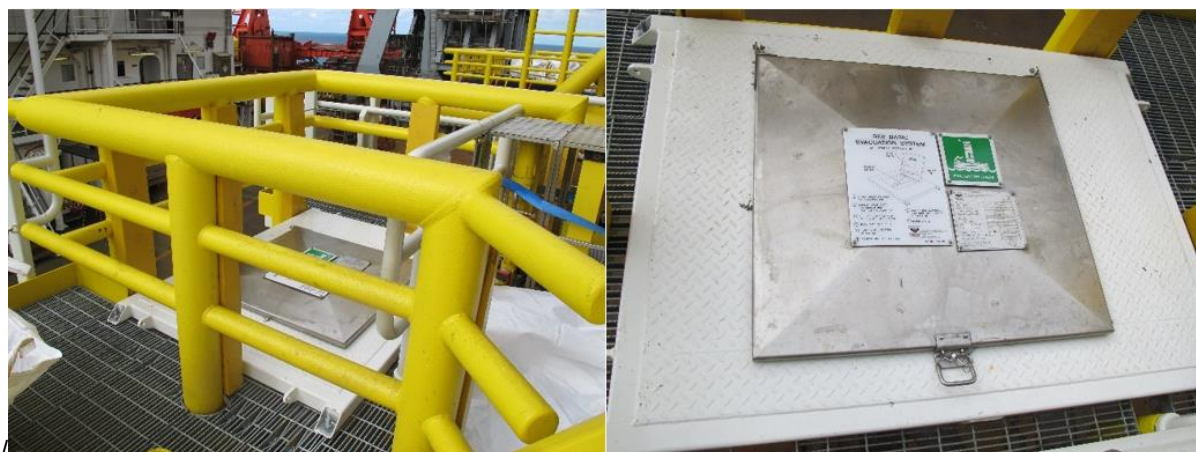
Figure 1. Example of escape chute arrangement
