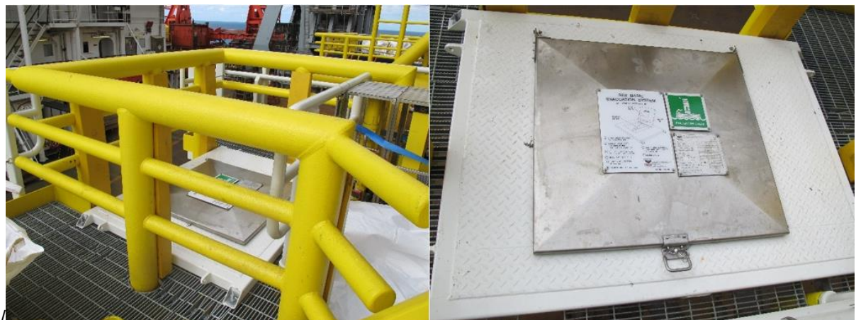
Figure 1. Example of escape chute arrangement
